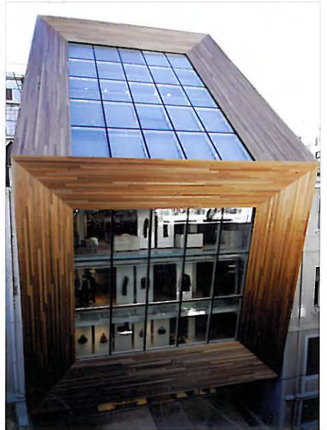
View of facade
